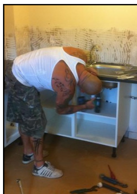
Garry, one of our contractors at work
